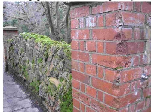
East end: London Clay beneath the weir from Jack's Lake; over-burnt bricks on the bridge over Pymms Brook coming from Jack's Lake – an indication of local brickmaking probably from the silty Claygate beds.
